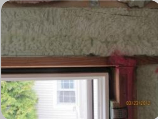
TERC 4.4.5 Advanced framing 4.4.5b All headers above windows & doors insulated
