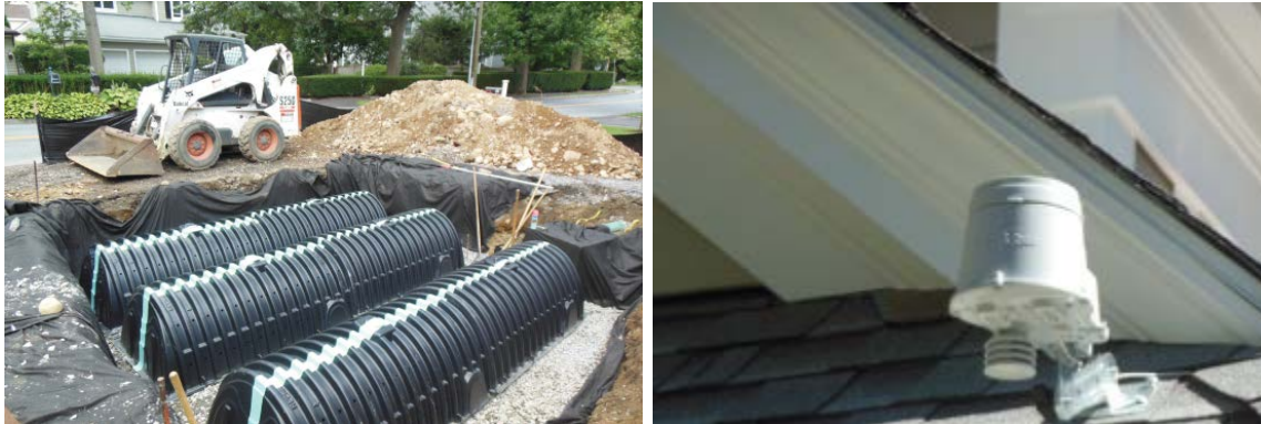
Figure 4. (L) Gallery system for gutter rainwater; (R) irrigation weather station (Preferred Builders Inc.)
