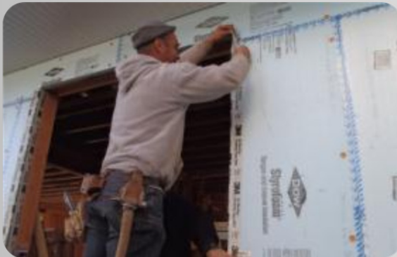
IAP Moisture Control- Water-Managed Wall Assemblies 1.6 Window & door openings fully flashed
