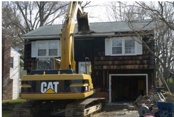
Figure 1. This 1970s home was taken down to make way for the “Performance House” (Preferred Builders Inc.)
