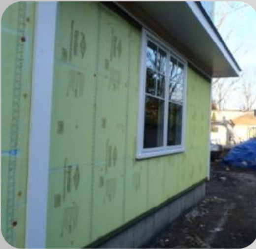
IAP Moisture Control- Water-Managed Wall Assemblies 1.5 Continuous drainage plane behind exterior cladding, properly flashed to foundation
