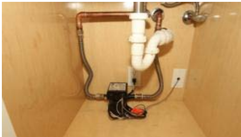
Figure 5. On demand pump under a bathroom sink (Preferred Builders Inc.)
