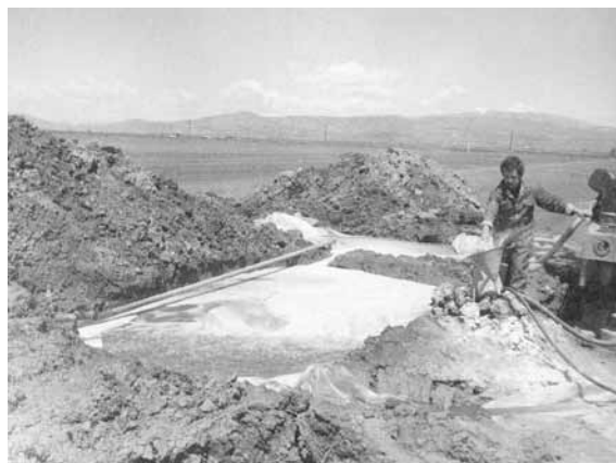
Example Photograph of a mud pit.
