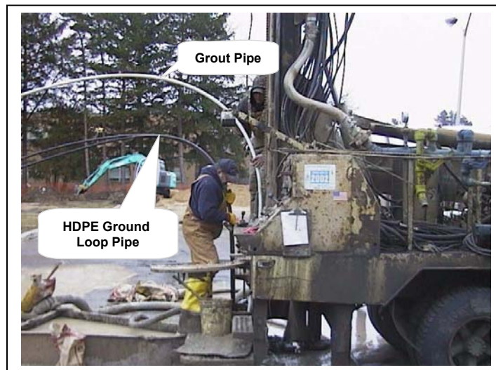
Figure 22 – Installing Pipe and Backfilling a Vertical Hole
