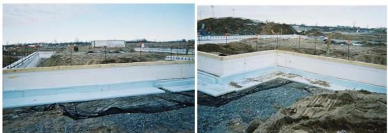
Figure 3 – Vertical and horizontal insulation
