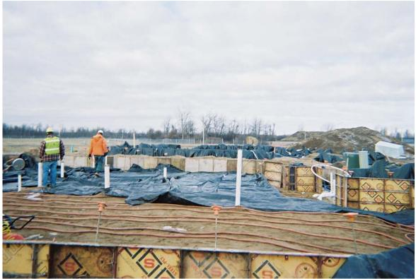
Figure 7 – Temporary tubing and covering used to keep slab area from freezing during construction
