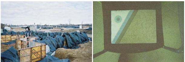
Figure 5 – Conventional concrete forms
